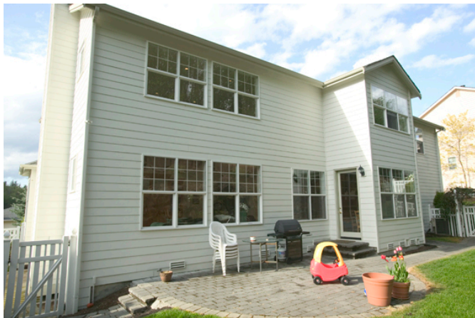
Camera is pointed up to get the top of the house in the photo
